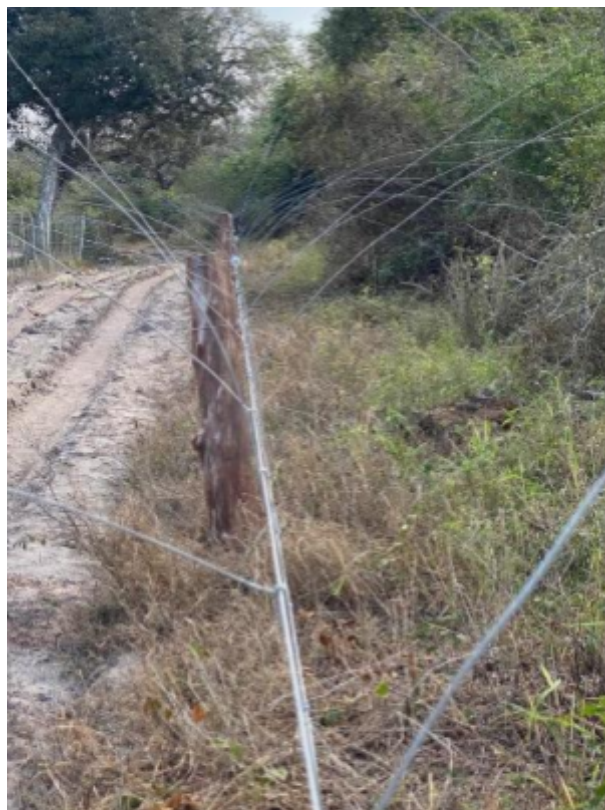
Figure . The newly designed and erected elephant 'proof', 'porcupine fence'
